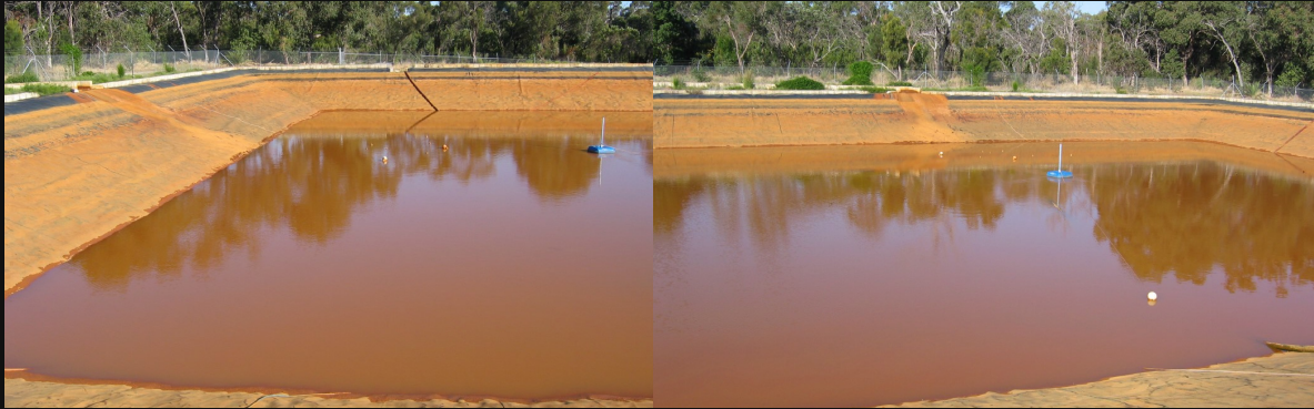
Concentration pond for Iron settlement. Note, Iron build-up on top of the sump in far-right image below. This indicates iron dropping out the water column from added aeration.
